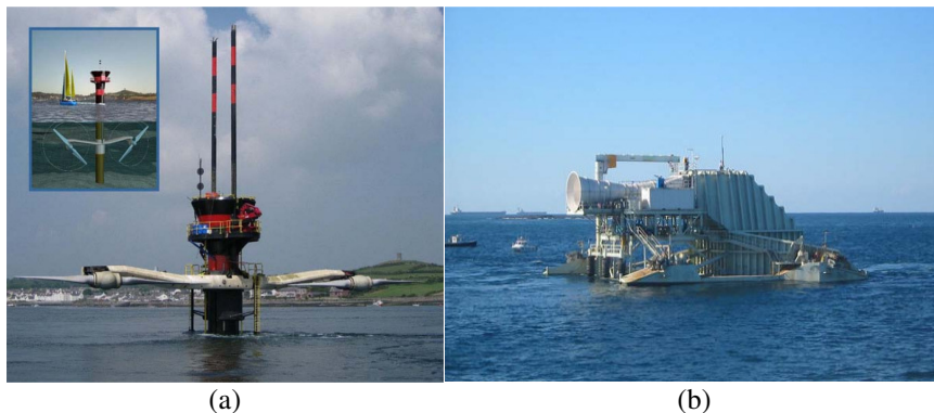
Figure 1-3: (a) Seagen, marine current turbine by Marine Current Turbines Limited [15], (b) oscillating water column by Oceanlinx [16]
